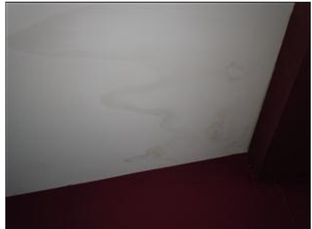
3.0 Picture 2 roof leak by chimney
