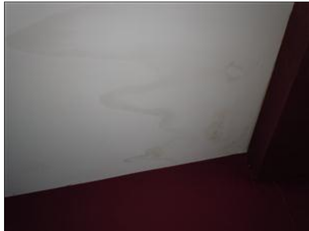
3.0 Picture 2 roof leak by chimney
